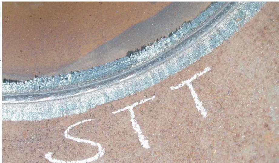
Figure 3. In side chamber view to weld joint root performed by STT welding process. The weld joint quality is on high level.
