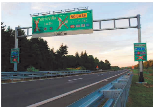
Figure 1. An example of supporting structure for placing traffic signalization
