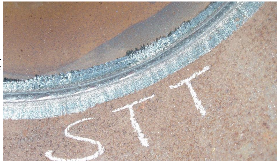
Figure 3. In side chamber view to weld joint root performed by STT welding process. The weld joint quality is on high level.
